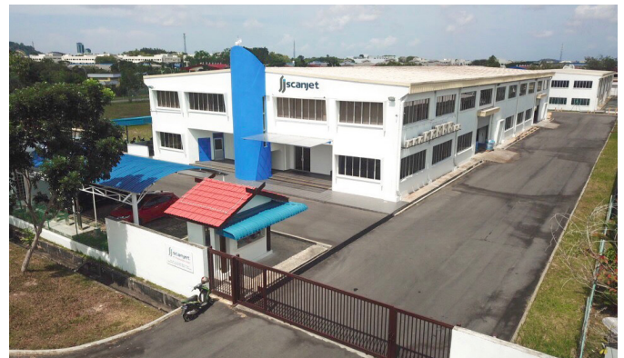
PT Scanjet Production Indah in Batamindo. Photo: Gabriel Brännlund
