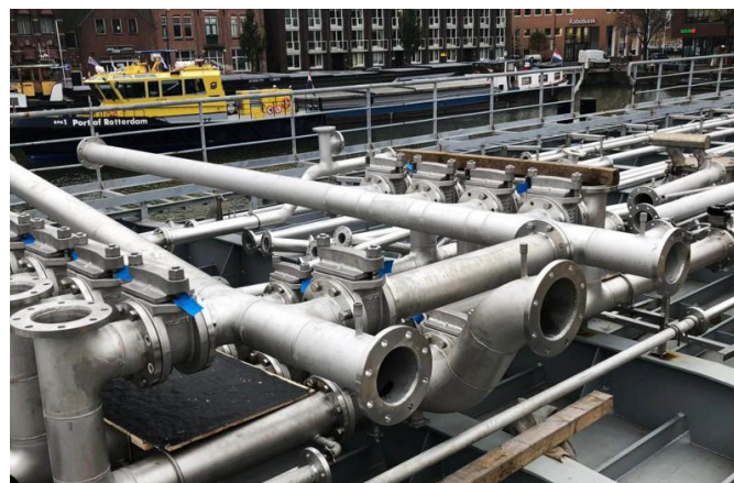
Nordic Flow Controls newly installed valves on a inland tanker in The Netherlands. A successful cooperation between Nordic and Maas Marine. Photo: Patrick Maas
