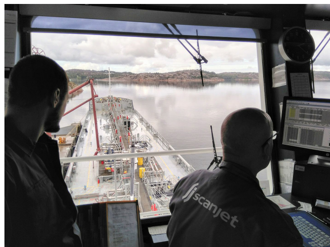
Scanjet Service Engineers during installation Photo: Unknown
