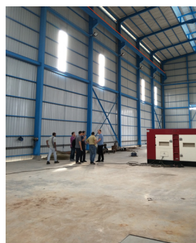
New factory in progress. -Batam, Indonesia.
