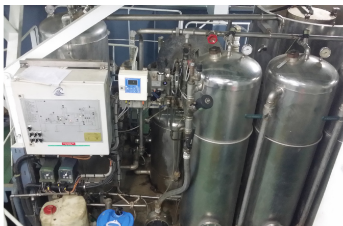
Scanjet service of MarinFloc waste water solution onboard Cruise Ship Sapphire Princess. Photo: Richard Santos
