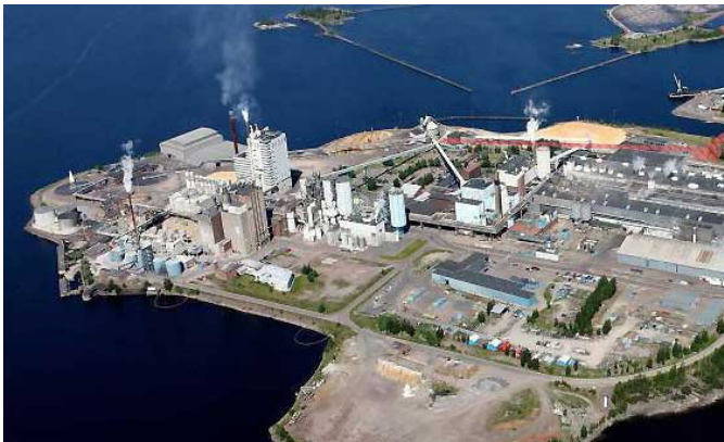
Stora Enso Paper Mill Factory in Skoghall, Sweden. Photo: Stora Enso.
